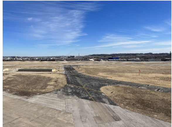
Taxiway D - East View
