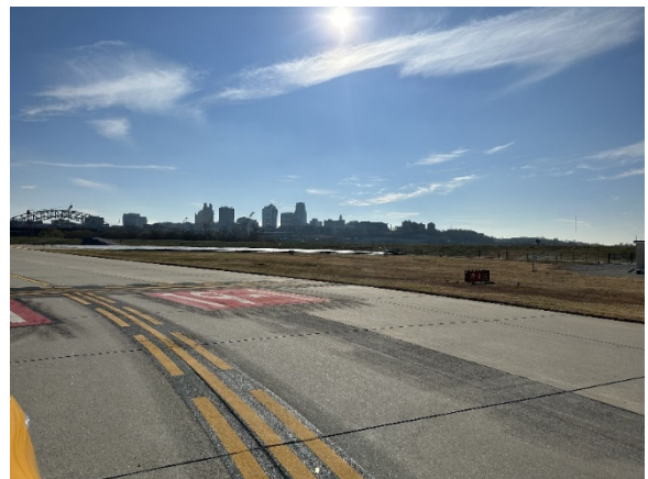
Pavement Markings (Enhanced Centerline, Runway Designation, & Holding Position)
