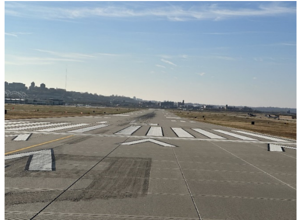
South View from Runway 19
