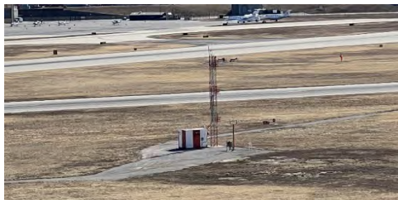
Glide Slope Antenna Serving Runway 4-22
