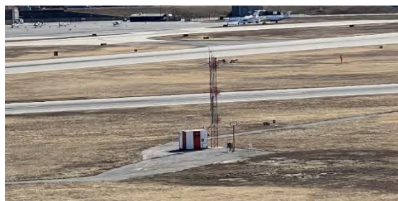
Glide Slope Antenna Serving Runway 4-22
